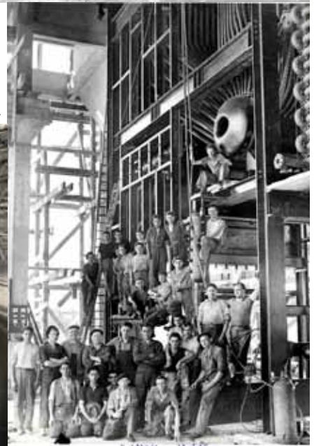
Panel production: A giant press formed steel panels for car bodies.
